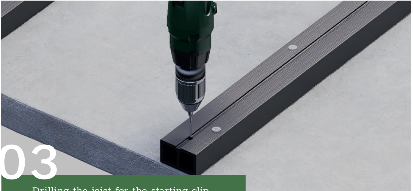
Drilling the joist for the starting clip
